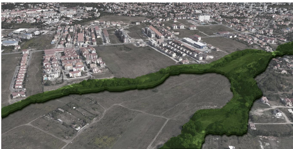
Figure 15. Aerial view of the area where we can see the indifferent relationship between the built environment and the watersheds present in the area.
